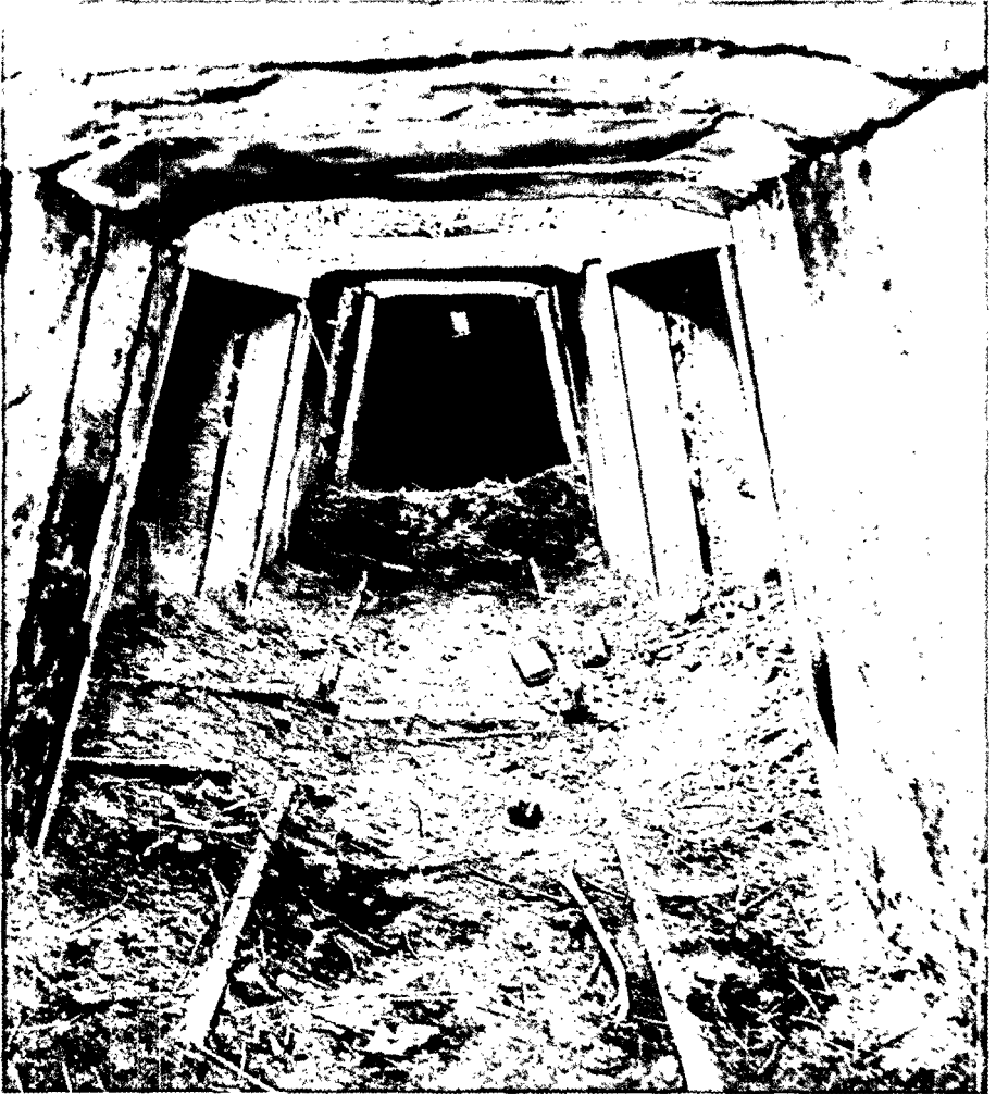
Inside of Underground DMZ Tunnel under Construction by North Korea
