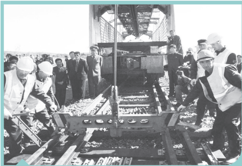
Modernizing railways between Rajin, North Korea and Hassan, Russia
